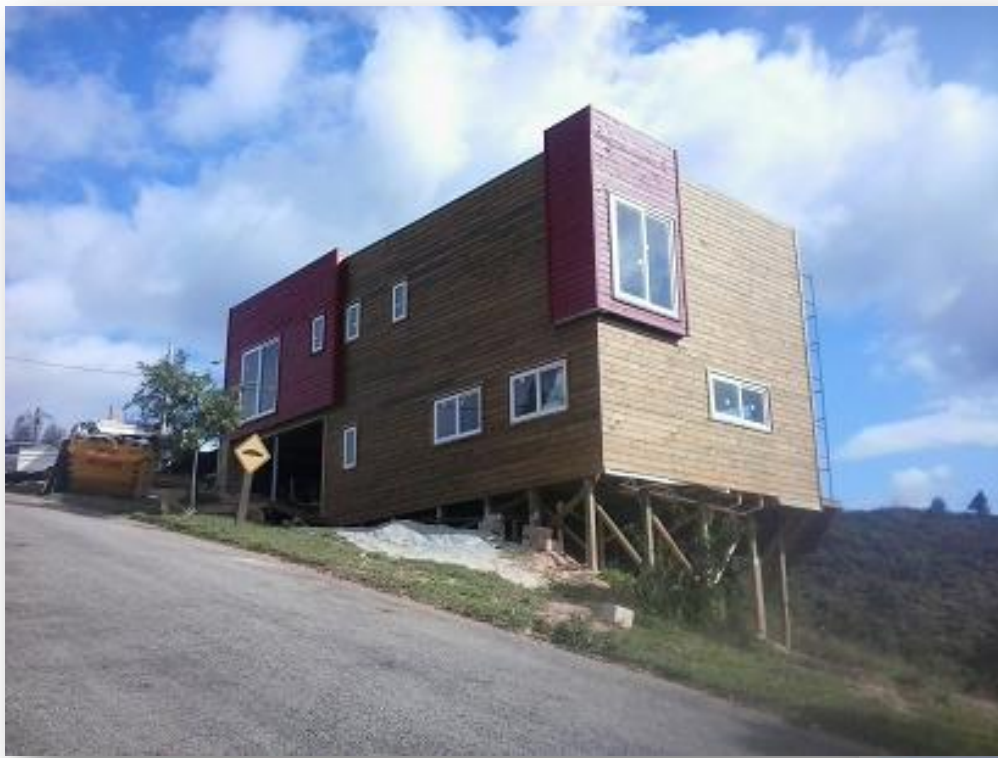
2012 - Condomínio Capital Ville - Cajamar/SP
